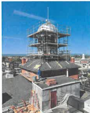
Modern reconstruction with PVC materials, a copper roof, restored chimneys, and bird protection
