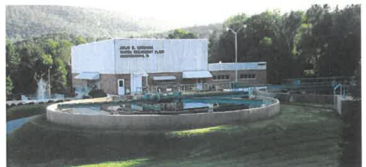
Chambersburg's Julio D. Lecuona Water Treatment Plant
