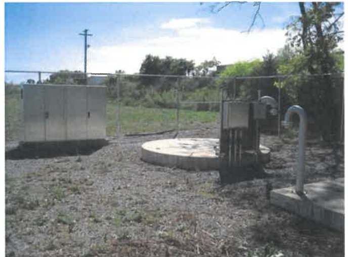
Typical Sewage Pump Station
