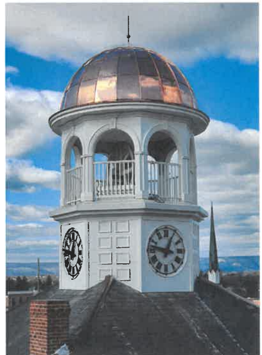
Clock Tower AFTER
