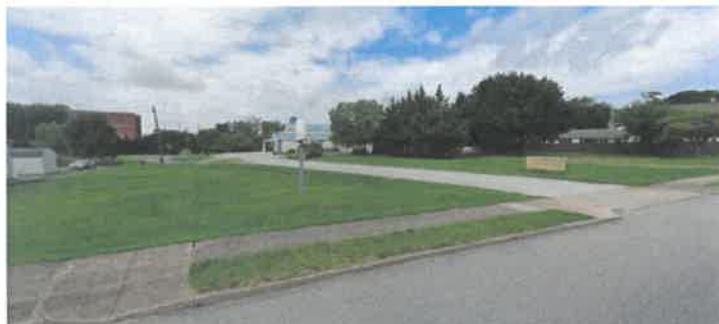
The Former Wagner Supply Depot is Owned by the Borough as is the House on the Right, Now Demolished, and the Cold Storage Building to the Rear, Scheduled for Demolition
